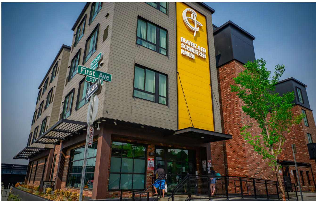
Schweitzer Haven is a 50-unit permanent supportive housing project owned and operated by Catholic Charities Eastern Washington. Onsite services include case management, access to primary healthcare, substance use and behavioral healthcare providers, and peer support. The building is located near Frontier Behavioral Health’s main downtown campus.
